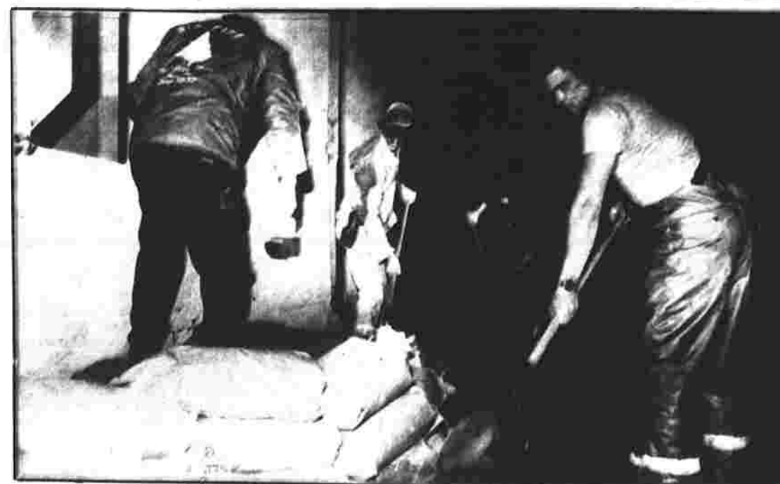
Residents and freighters from Westfield, Wis., fill sandbags in low-lying areas Tuesday in anticipation of a dam bursting about three miles away. About 200 people were evacuated.
